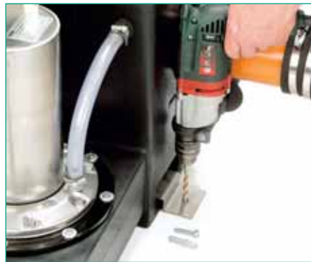
Assembly anti-buoyancy safeguard
